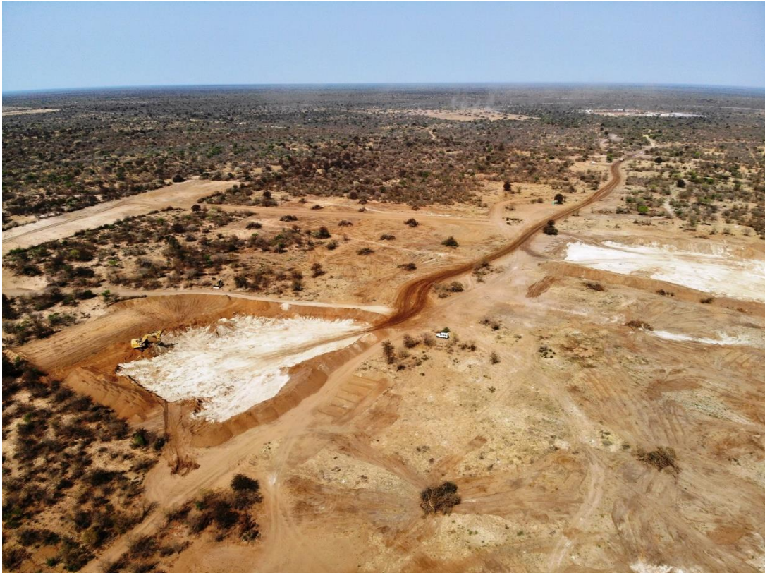
Figure 1: Clearing of topsoil T3 Stage 1 Open Pit and for the process plant and accommodation village in the background.
